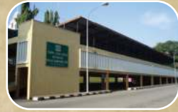
14. Municipal Car Park
